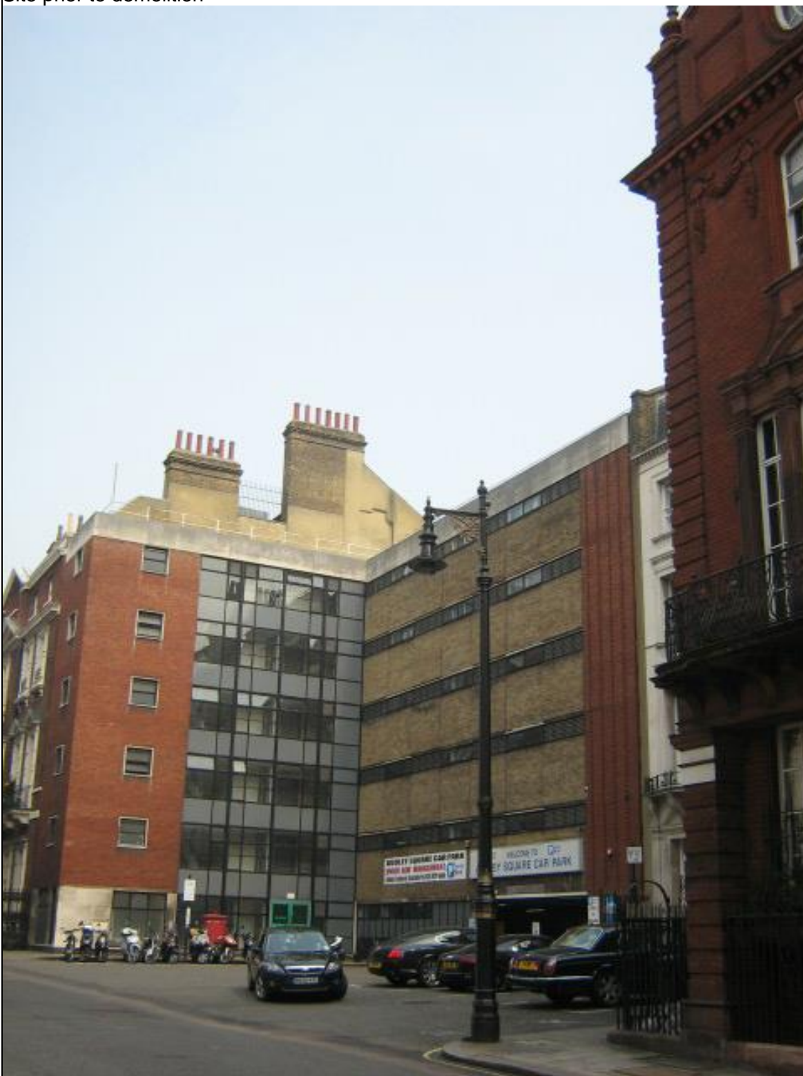
Site prior to demolition
